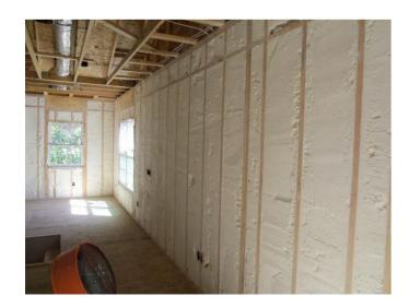
Closed Cell 2 lb. Foam –Excellent Insulating Properties. Closed cell 2 lb. foam is sprayed onto walls as a liquid before expanding into a hard foam. Closed cell foam is completely air tight, moisture proof, guaranteed for the life of the home owner and actually adds strength to the building it is installed in.
